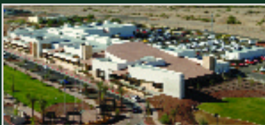
CITY OF SURPRISE PUBLIC SAFETY BUILDING
